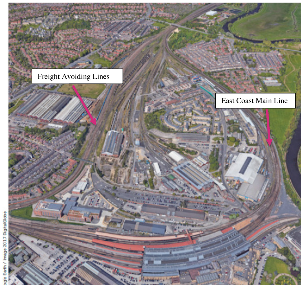
Figure 1: Aerial Image of the York Central Site
